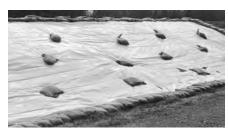
laid out flat on the slope, sandbags are placed around the perimeter with additional bags placed randomly for weight. If the slope is steep, wooden stakes can be driven into the ground just above the area to be protected. The stakes are 4 feet apart with a 1-foot stagger. The plastic is secured to the stakes with tie-down buttons or small round rocks (see Figure 13).
